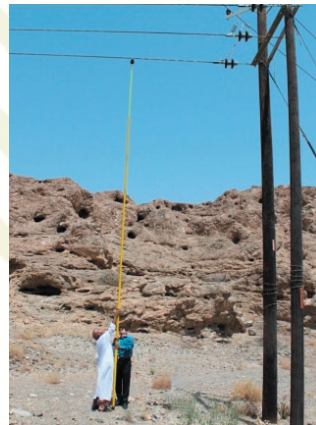
figure 7 - installation with a telescopic hotstick
